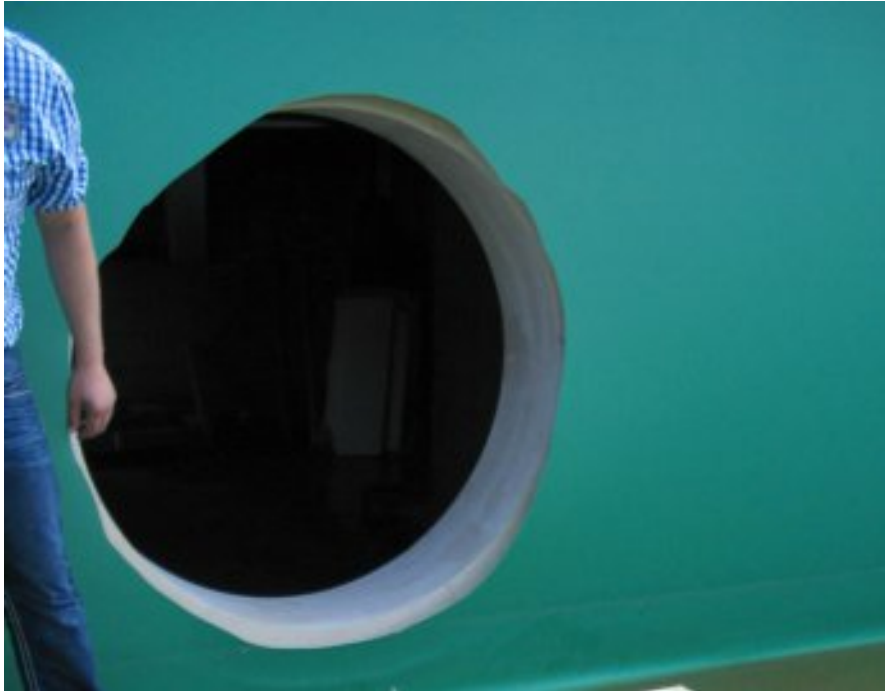
Abbildung 3: The picture shows a foto with the round opening. The green liner on top of the concrete opening is already prepared.
