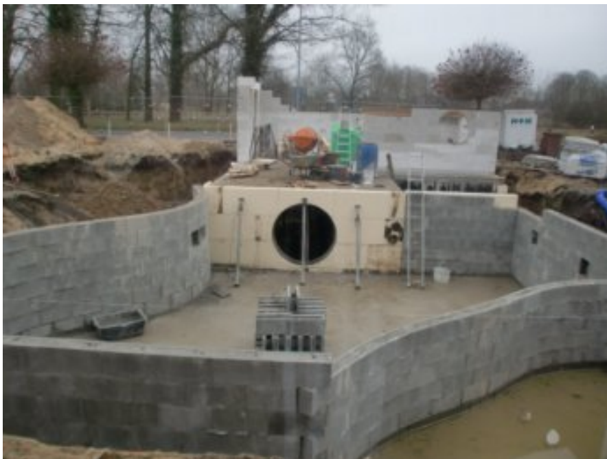
Abbildung 2: Pool beeing build, circular wall opening beeing prepared
