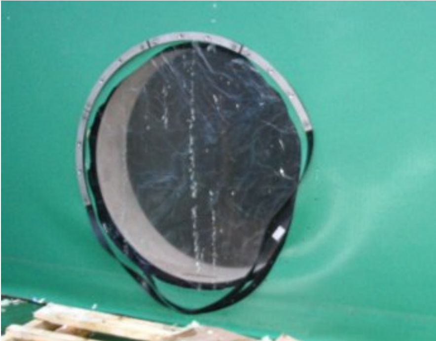
Abbildung 11: One rubber between liner and acrylic block (rubber 2). One rubber between liner and steel blind (rubber 1). Steel blind on top. Fasten all starting at the top of the window.
