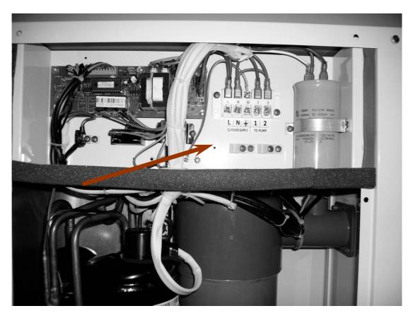
Remark – For models with 3 phases, switching 2 phases may cause an inversion in the rotational direction of electrical motors, which could damage the unit. Therefore, a protection device has been built in, which will interrupt the circuit if the connection has not been performed correctly. If you see a red LED light up at the top of this protection device, **2 phase wires have to be switched**.
